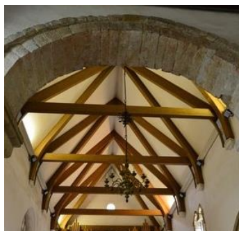
The roof - made simpler and lighter following the fire which destroyed the 1870 Victorian structure
