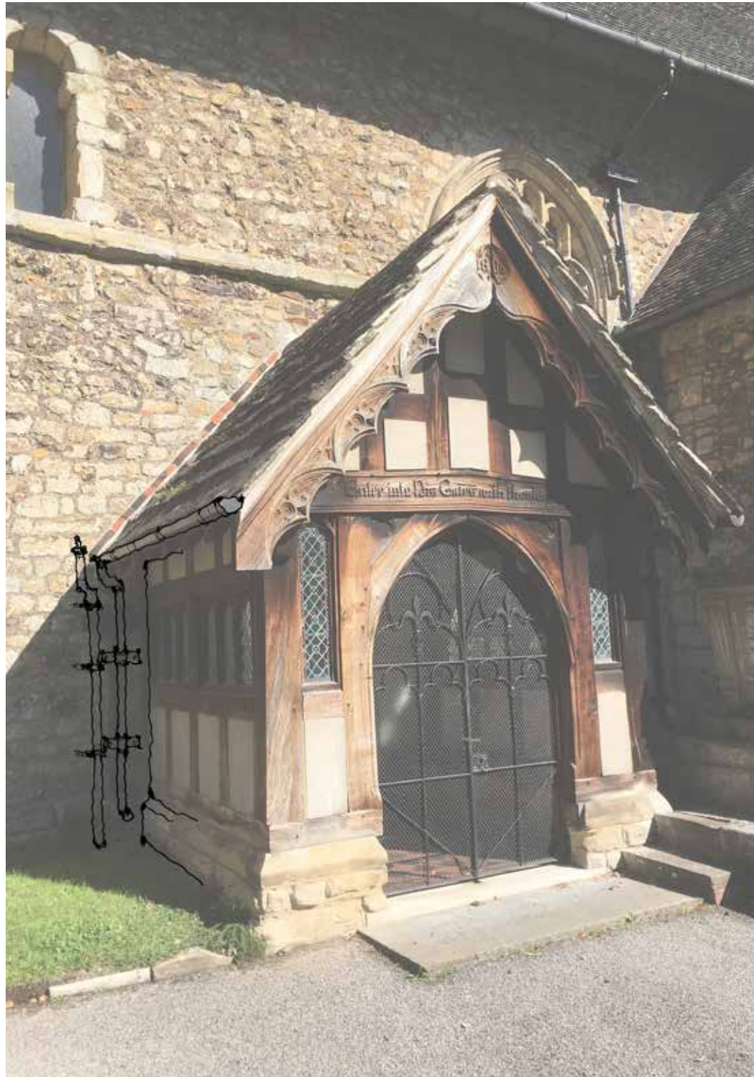
Fig 30: Proposed soil vent pipe serving macerator. Proposed to be discreetly mounted adjacent to existing rainwater downpipe.
