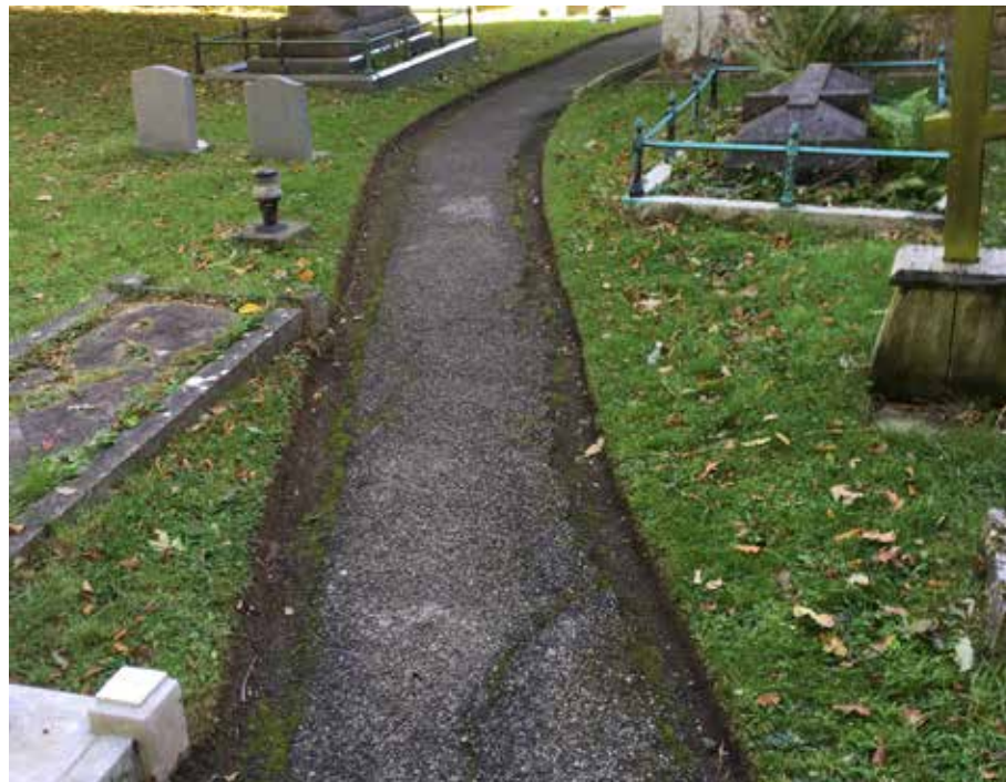
Fig 8: Photograph of a section of cracked tarmac pathway around the periphery of the church.
